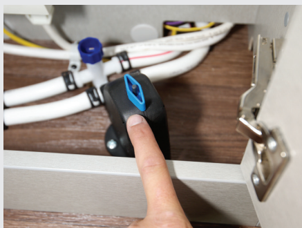
This automatic boiler valve will trigger and dump your boiler water at 4°C
