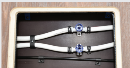
Before draining out all of the water, ensure stopcocks and valves are open
