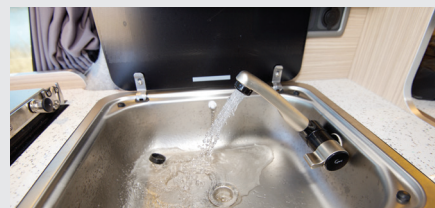
When recommissioning the 'van water system, clear air from pipes by opening tap furthest from the fresh-water tank and keep open until it stops spitting
